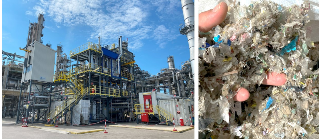
Figure 4: Pilot plant of OMV reoil-process and typical input material.
